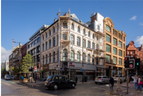
View K: Existing View
